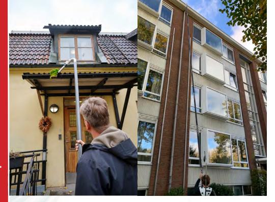
Our External Cleaning System is a simple, durable system for the cleaning and maintenance of guttering and downpipes capable of reaching up to a height over 10 metres from the safety of the ground floor.
